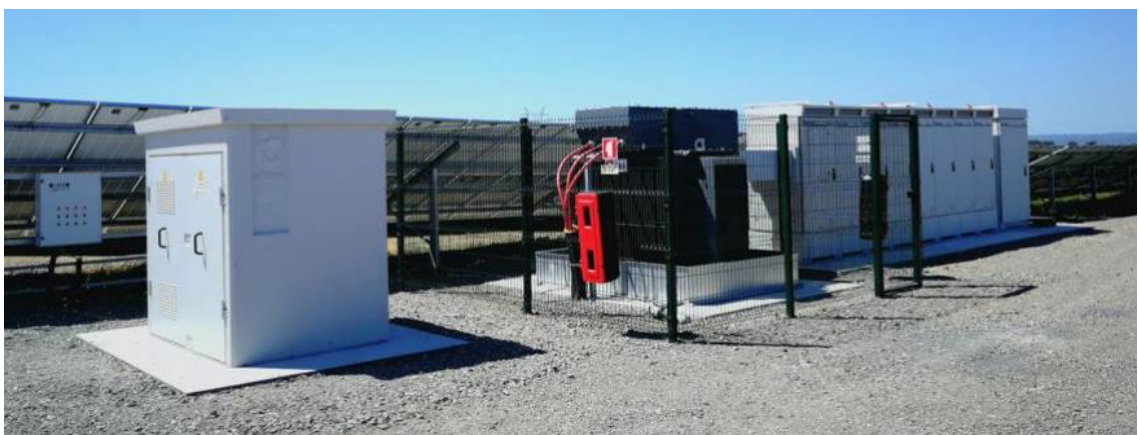
Insert 4-6 Typical Disaggregated Conversion Unit
